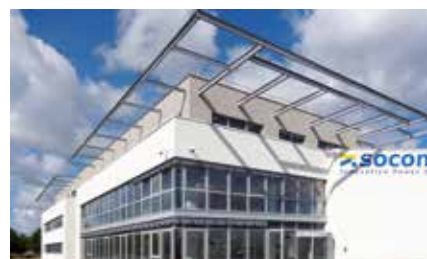
Socomec Green Building.
