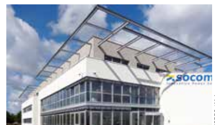
Socomec Green Building.
